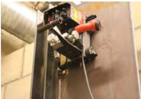
Vertical fillet welding
