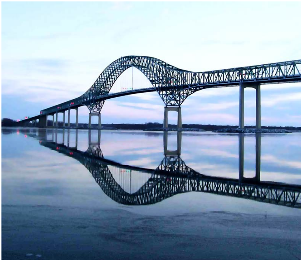
Lavolette Bridge over the St. Lawrence River.
