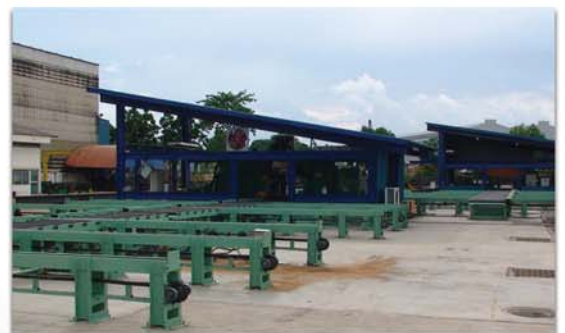
Peddinghaus users commonly employ garage style structures outside of their main welding and fabrication shop.
