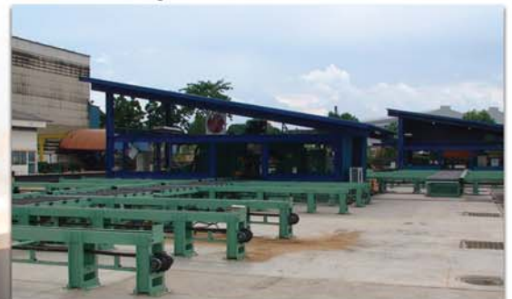
Peddinghaus users commonly employ garage style structures outside of their main welding and fabrication shop.
