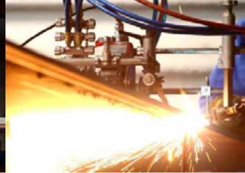
Chamfering (1:4 ratio beveling) using single torch
