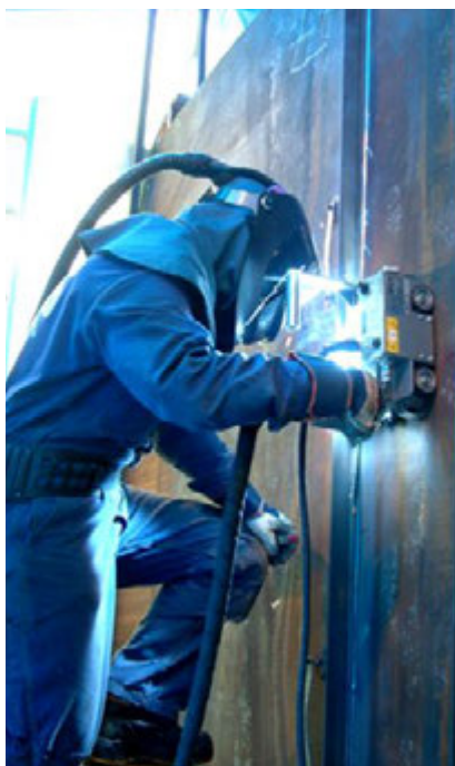
Vertical up butt welding using guide rail
