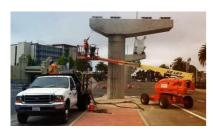
**Outdoor/urban environments.** Dry blasting requires substantial containment/tenting to maintain airborne dust levels within legal limits. In outdoor and urban environments, such containment is not practical or cost-effective. Due to inherent dust suppression, **vapor abrasive blasting operations require minimal containment.**
