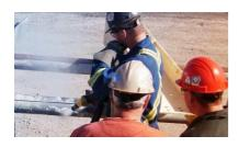
**Alongside other workers.** Dust from dry blasting presents not only an inhalation health hazard, but severely limits visibility. Whereas dry blasting operations must be sequestered from normal operations, **wet blasters can work in close proximity with other workers with minimal precautionary measures**.
