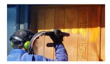
**Delicate surfaces.** Wet blasters can operate effectively at lower PSI, **removing coatings without damaging the underlying substrate.** Vapor abrasive blasting is a preferred method for blasting antique, fragile surfaces and soft surfaces (including wood). In addition, the presence of lubricating water reduces heat due to friction that can warp metal surfaces.
