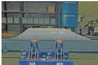
Adjustable supports to level pipe at cut location.
