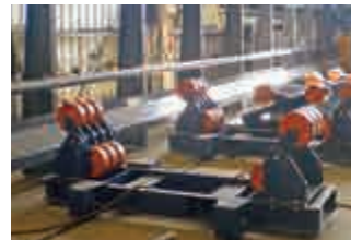
Heavy load supports to level 4000 mm OD pipe at cut location.
